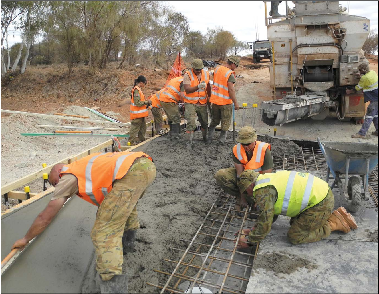
The AACAP Construction Troop from the 21 st Construction Squadron work with civilian equipment to mix high volumes of concrete necessary for culvert bases.
