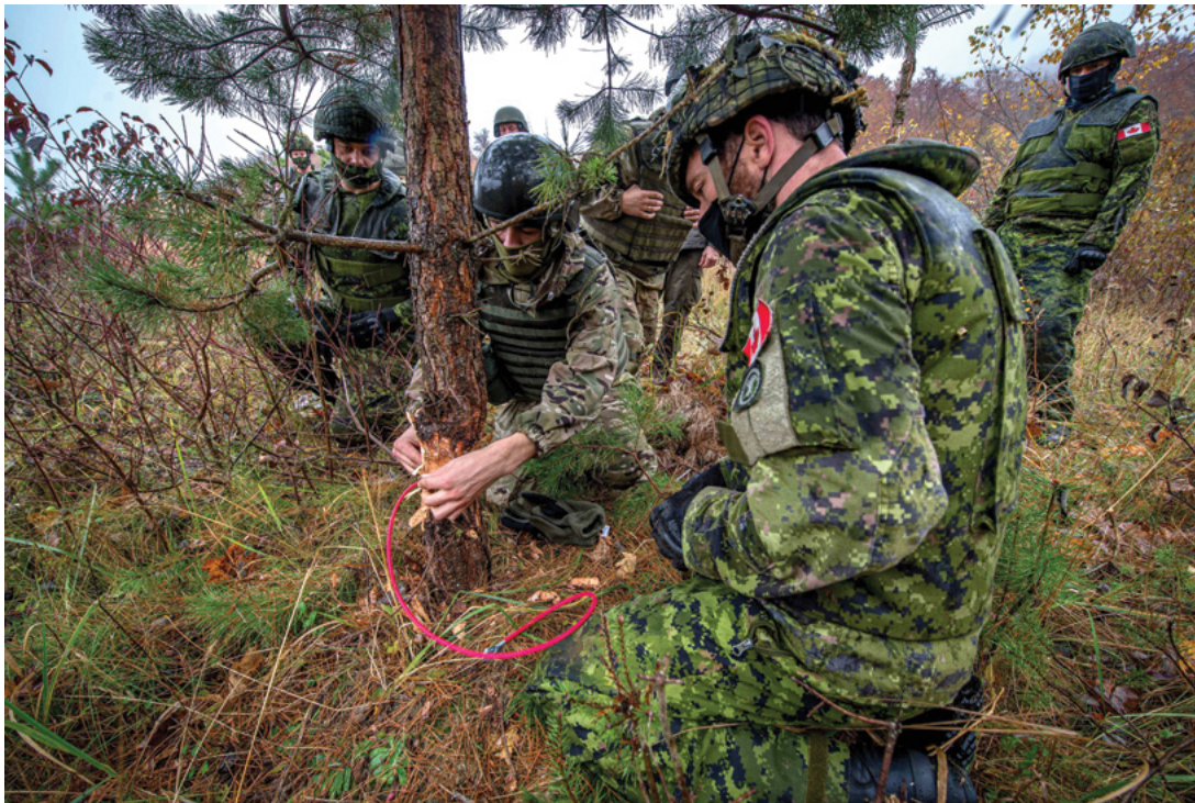
The Roto 10 Operation UNIFIER Engineer Development Team (EDT) advises the National Guard of Ukraine (NGU) in demolitions ranges as part of Sapper Level 1 Training, 3 November 2020, in Zolochiv Ukraine.
