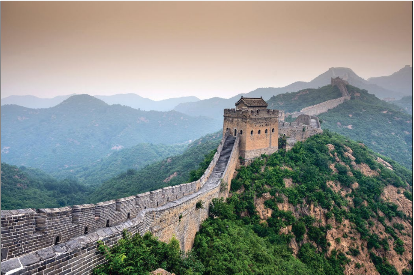
The Great Wall of China.
