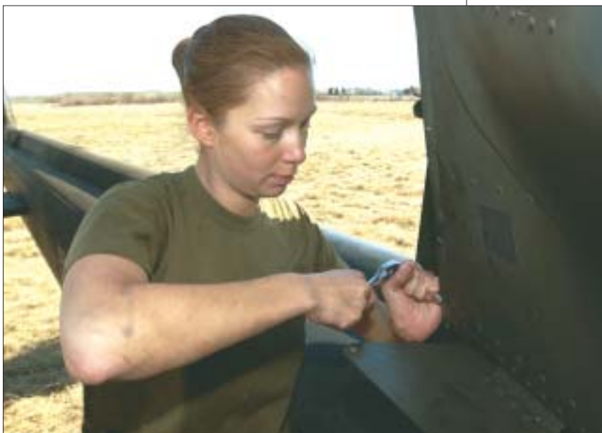
Repairing a Griffon helicopter belonging to 408 Tactical Helicopter Squadron during the Army’s first major field exercise of the century, Camp Wainwright, April 2003.
