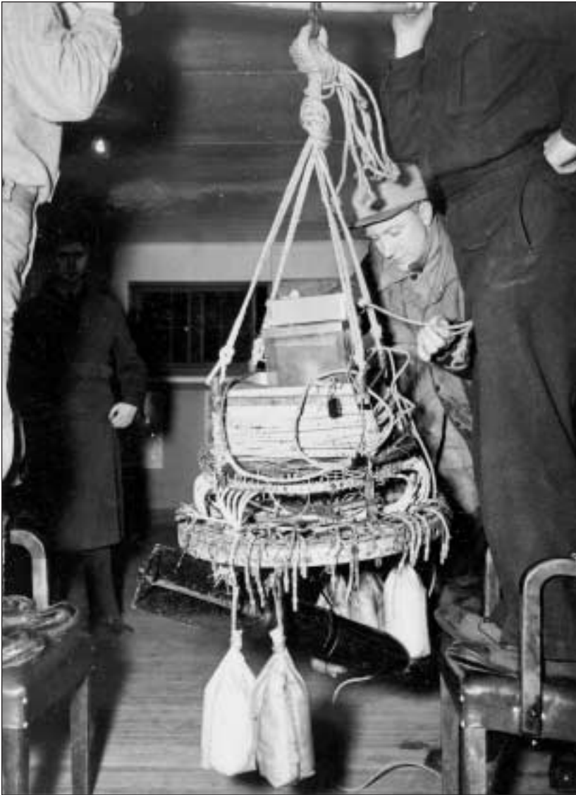
The chandelier, as the underslung carriage was known, from the balloon forced down near Coal Harbour was recovered intact. The picture shows the overall size of the sandbags and equipment carried by the balloon. It also includes the small battery target at which RCAF pilots were instructed to shoot to bring down a balloon intact.
