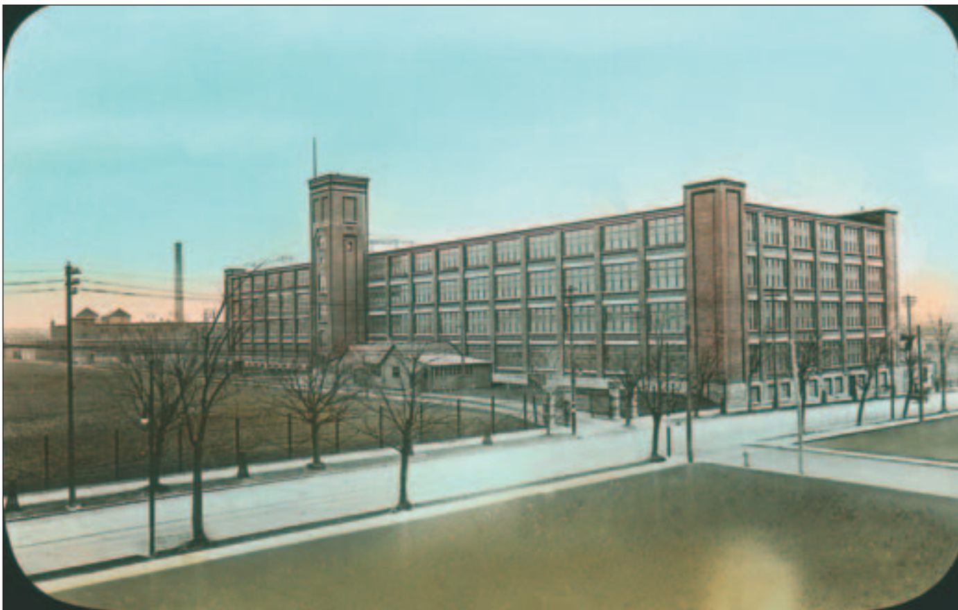
The Wabasso Cotton Company mills in Three Rivers, Quebec, circa 1930. The building was previously the militia armouries.
