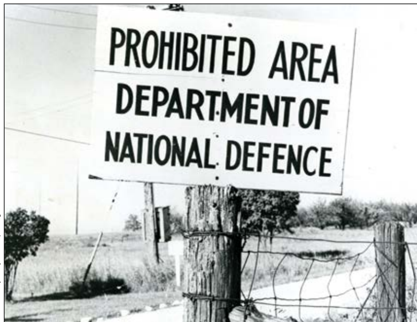
Keep out sign at the wartime entrance to Camp X.
