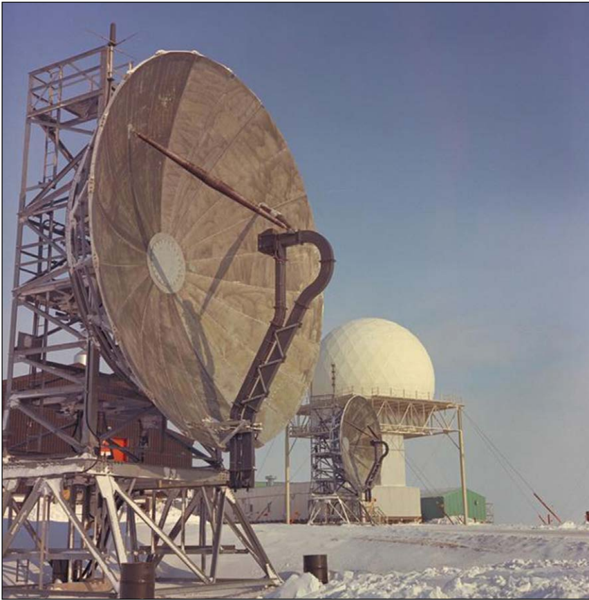
Close up of a radar antenna with the dome in the background. This DEW Line site is located at Cambridge Bay in the Arctic.
